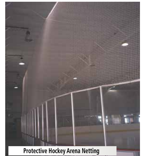
Spectator Protective Netting
